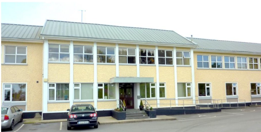
Figur 79 Indgang Dairy Research Centre's auditorium. Animal & Grassland Research and Innovation Centre, Teagasc, Moorepark, Fermoy, Co. Cork, Ireland. http://www.teagasc.ie
